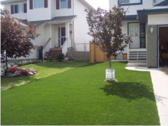
Incorrect – There should be a distinct boarder installed between the artificial turf and the neighboring natural sod.
