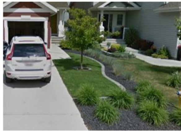
Correct – A distinct boarder containing additional shrubs has been installed between the artificial turf and neighboring sod.
